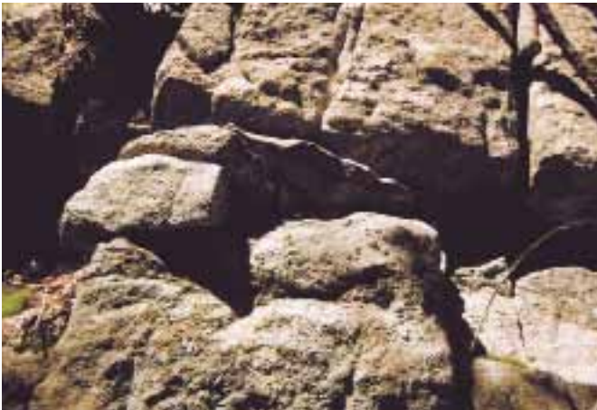
Crumbling and excessively fractured rock face
