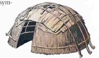
A wigwam made of grass mats tied to saplings and covered with slabs of bark
