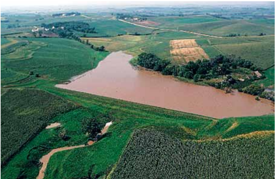
Watershed dams like this one in Iowa help control runoff from streams and hold and store sediment.
