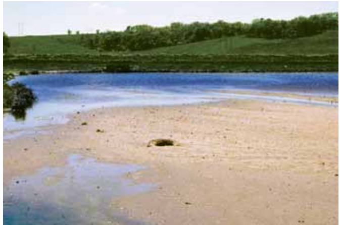
In large amounts, such as caused by accelerated erosion, sediment can be a pollutant and create costly problems. This small reservoir is rapidly becoming filled by sediment.
