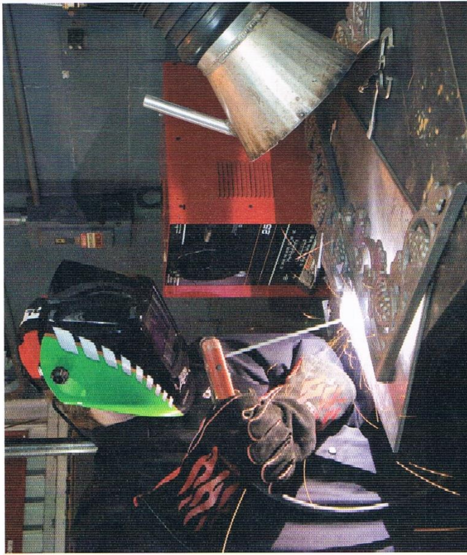
Welder using shielded metal arc welding
